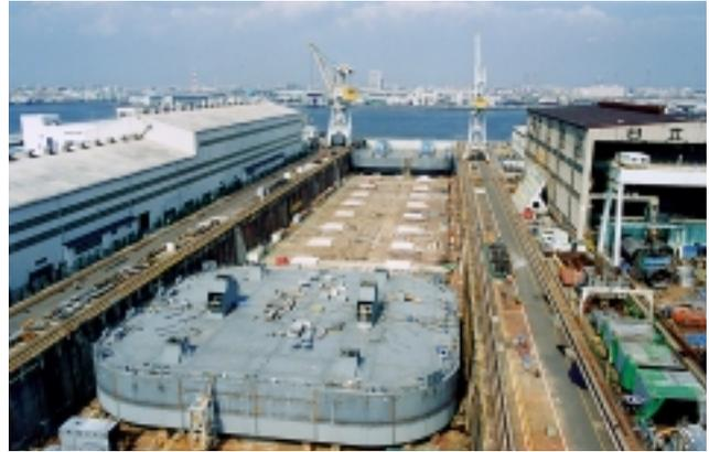
Photo 6 Pontoons Installed
