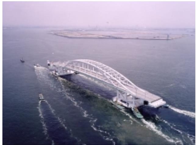
Photo 11 Floating Bridge Is Being Towed
