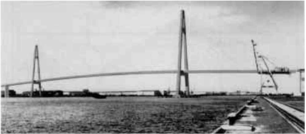
Fig. 3. Nagoya Harbour Bridge, Japan.
