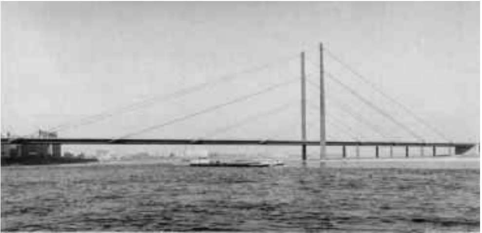
Fig. 16. The slender free standing towes of Kniebrücke in Düsseldorf, West Germany.
