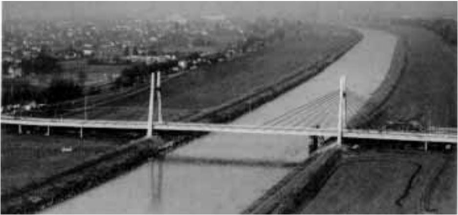
Fig. 25. Bridge across the Rhine at Diepoldsau, West Germany. Span = 97 m (318 ft).
