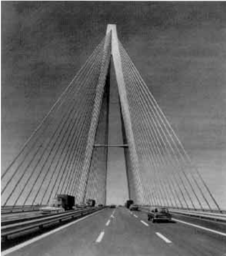
Fig. 20. View of A-shaped tower as motorist approaches bridge. There is an inherent feeling of comfort and safety.
