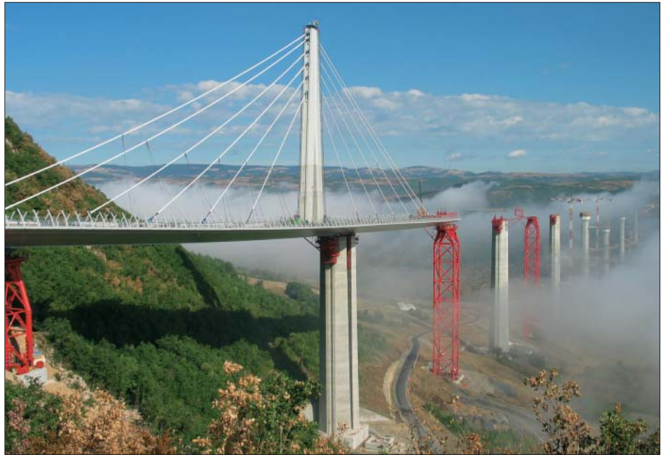
Fig. 7: Launching of girder with front pylon and cables in place
