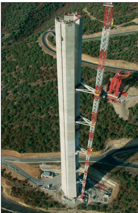
Fig. 6: Tower crane used to construct piers
