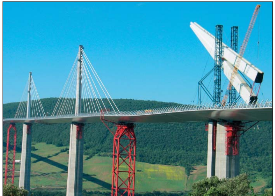
Fig. 10: Pylon being tilted up into position
