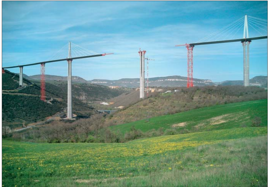
Fig. 8: Launching operations nearing completion
