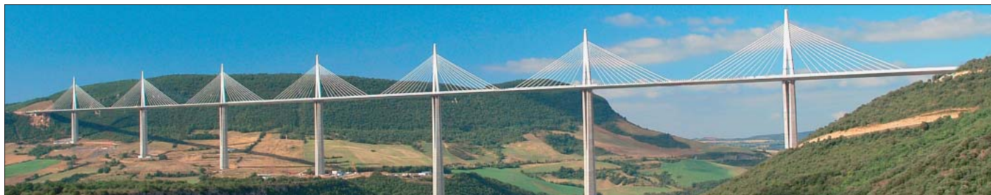
Fig. 1: View of Millau Viaduct near completion (Photo: Phototheque Eiffage/D. Jamme)
