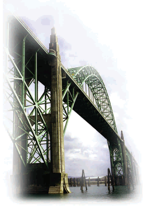
Highway Bridges Along US 101 The Pacific Coast Scenic Byway
