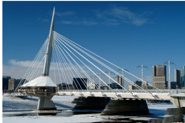
Esplanade Riel Bridge, Winnipeg (Source: City of Winnipeg)
