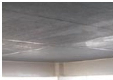
栈橋下面埋設型枠としての利用 Application for Floor Slab of Jetty Structure (lower surface)
